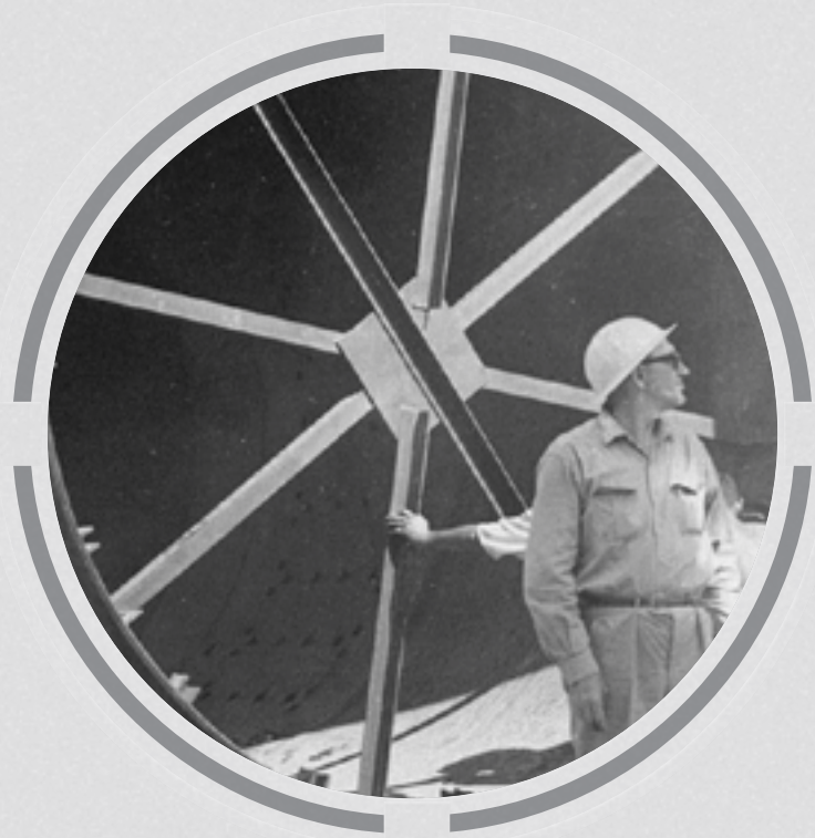
CONSTRUCTION OF THE FIRST PLANT IN SANTA HELENA, BRAZIL
